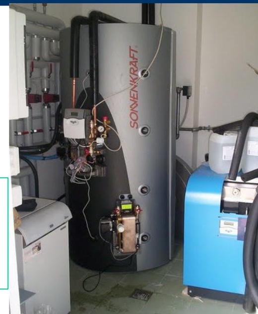
**Solar conditioning with high solar fraction and integration with heat pumps in Milan**
