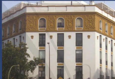
Solimpeks Solar SL, Seville, Spain
